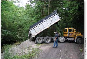
Limestone sands dumped into tributaries of the Cheat River help neutralize acidic waters in the stream and in the lake downstream.
